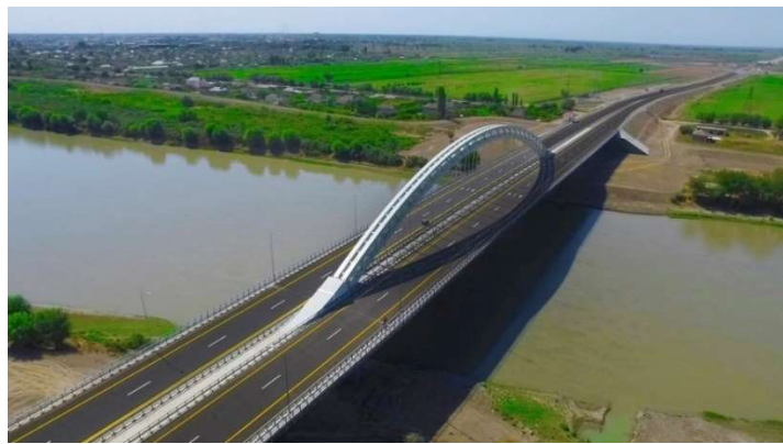
Picture 1. The newly constructed bridge [6]
