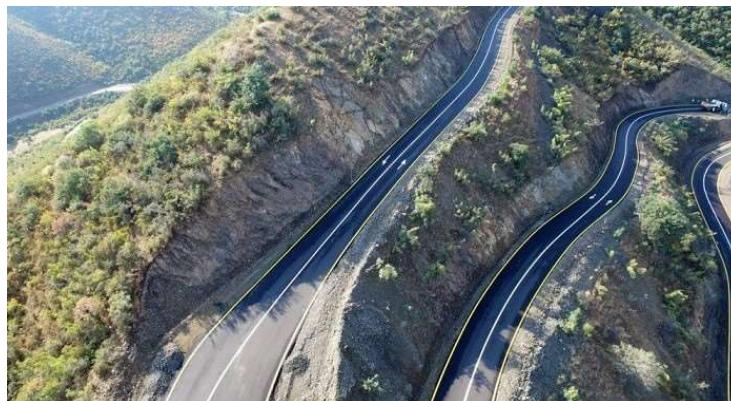
Figure 3. Modern road construction [2]
