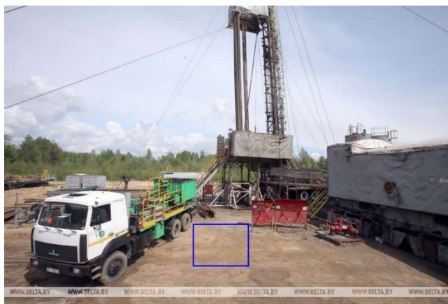
Fig. 20. Photograph of the drilling rig location at the Izbryn oil field [21].
