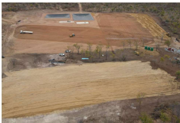
Fig. 13. Photograph of the Mukuyu-2 well drilling site [4].
