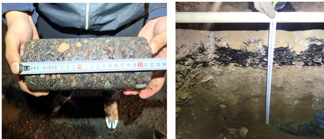
Fig.2 – opening the roadbed
