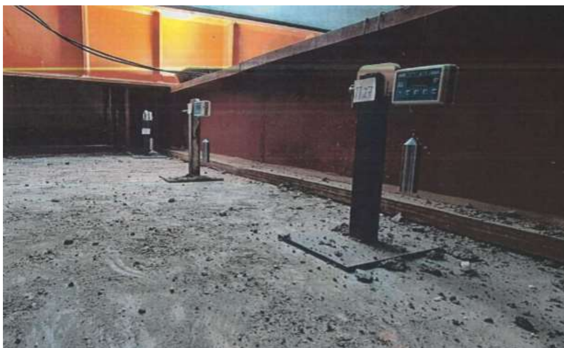
Figure 2.15 -Photo of MG-4 vertical deflection meters under the stylobate
