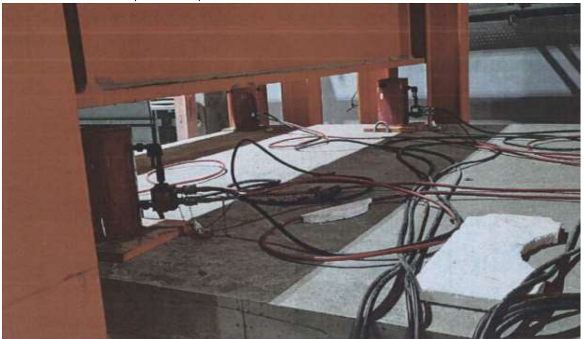
Figure 2.11 - View of the hydraulic jacks location area in the power stand.
