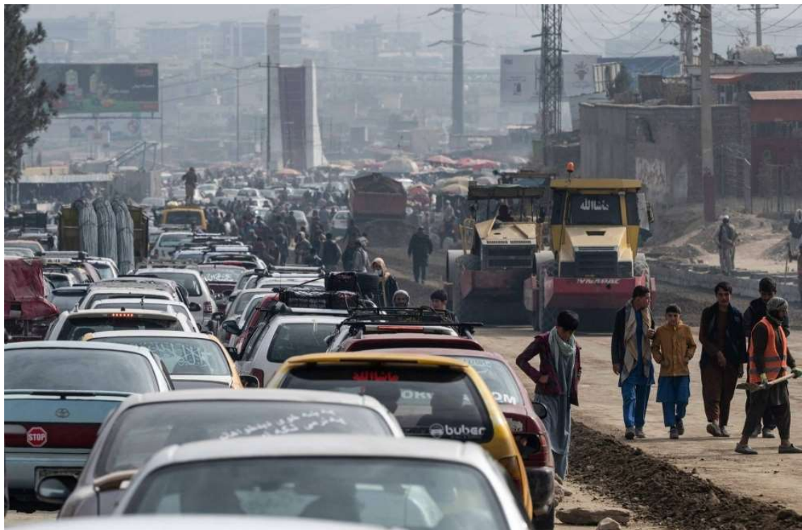
Commuters in Kabul make their way through traffic as construction laborers work on a road on Nov. 21
