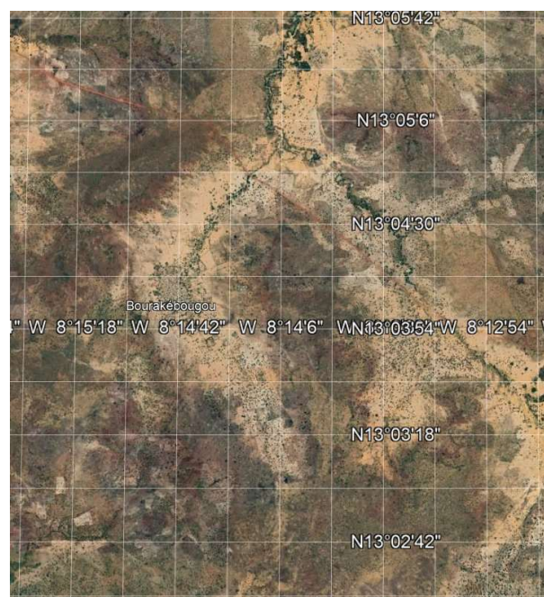
Fig. 29. Satellite image (Google Earth) of a hydrogen production site in Mali.
